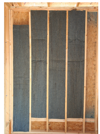
Just like a blanket to work with, the fiber composition makes for easy tearing and cutting. It's easily sized for hard to reach places.
