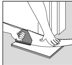
If a door frame needs to be cut, use a piece of plank to obtain the correct height.
